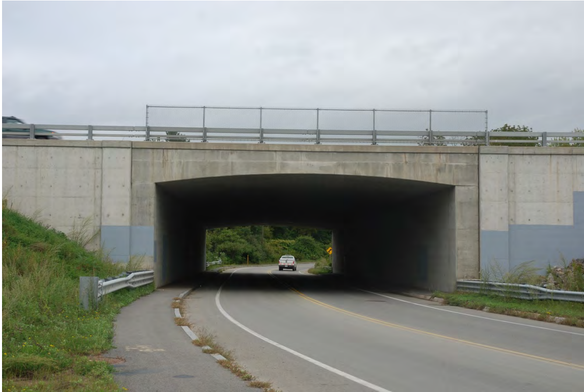
Photo # 33 Description: Spaulding Turnpike Bridge over Shattuck Way (Newington 103/124)
