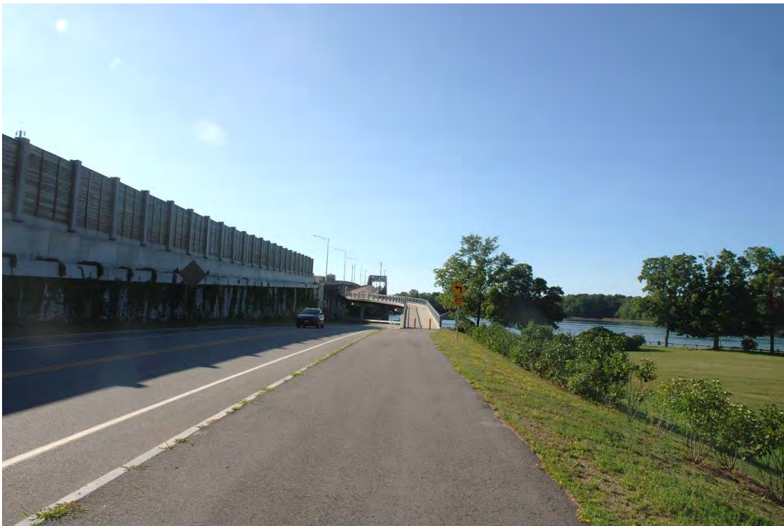
Photo # 18 Description: View along Hilton Park Road toward General Sullivan Bridge approach, Hilton Park Roadside Safety Rest Area (“Hilton Park”) on right
