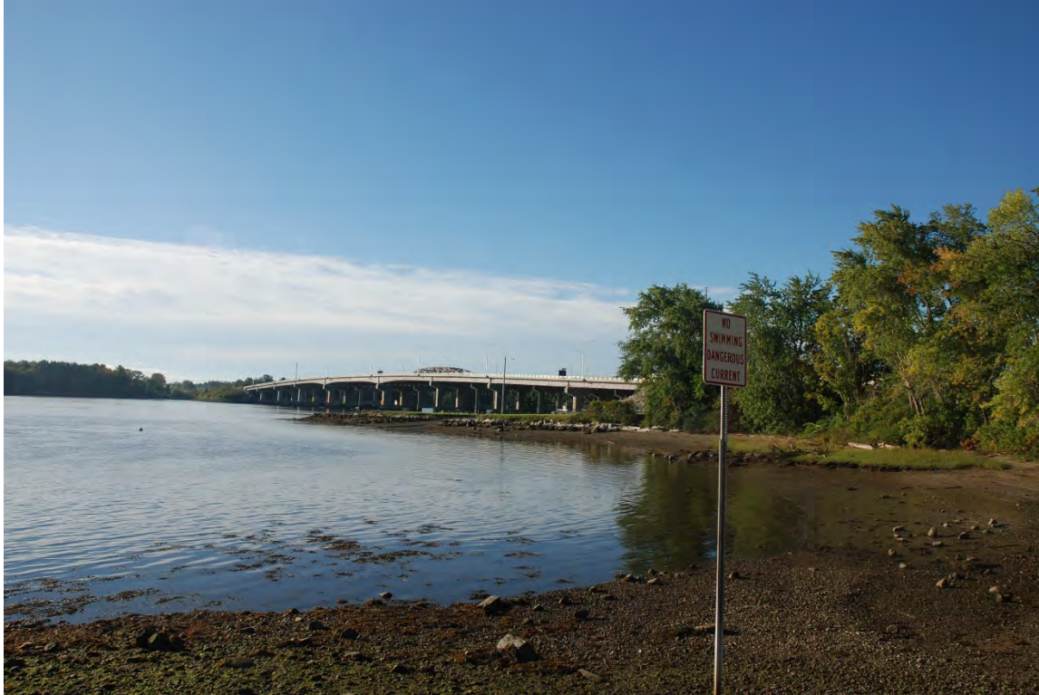
Photo # 23 Description: View of Little Bay Bridges and General Sullivan Bridge from Hilton Park east side Reference (file name or frame #): 23_11238S Direction: S Date: Sept. 2018
