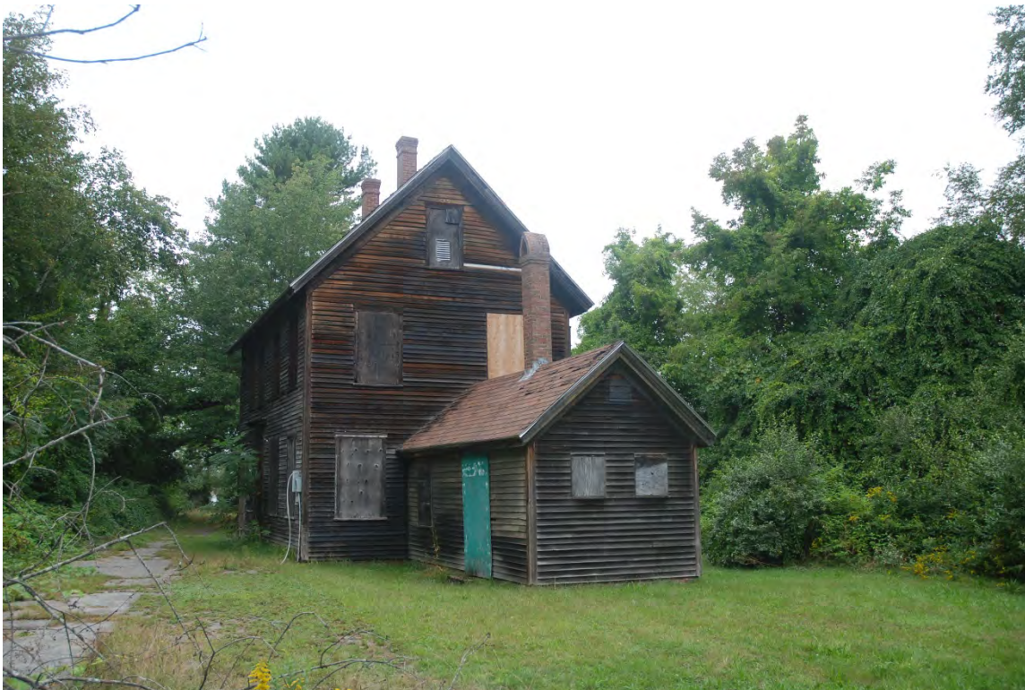
Photo # 30 Description: Newington Railroad Depot and Toll House, 24 Bloody Point Road, NWN0168 (NR-listed) Reference (file name or frame #): 30_11238S Direction: N Date: Sept. 2018
