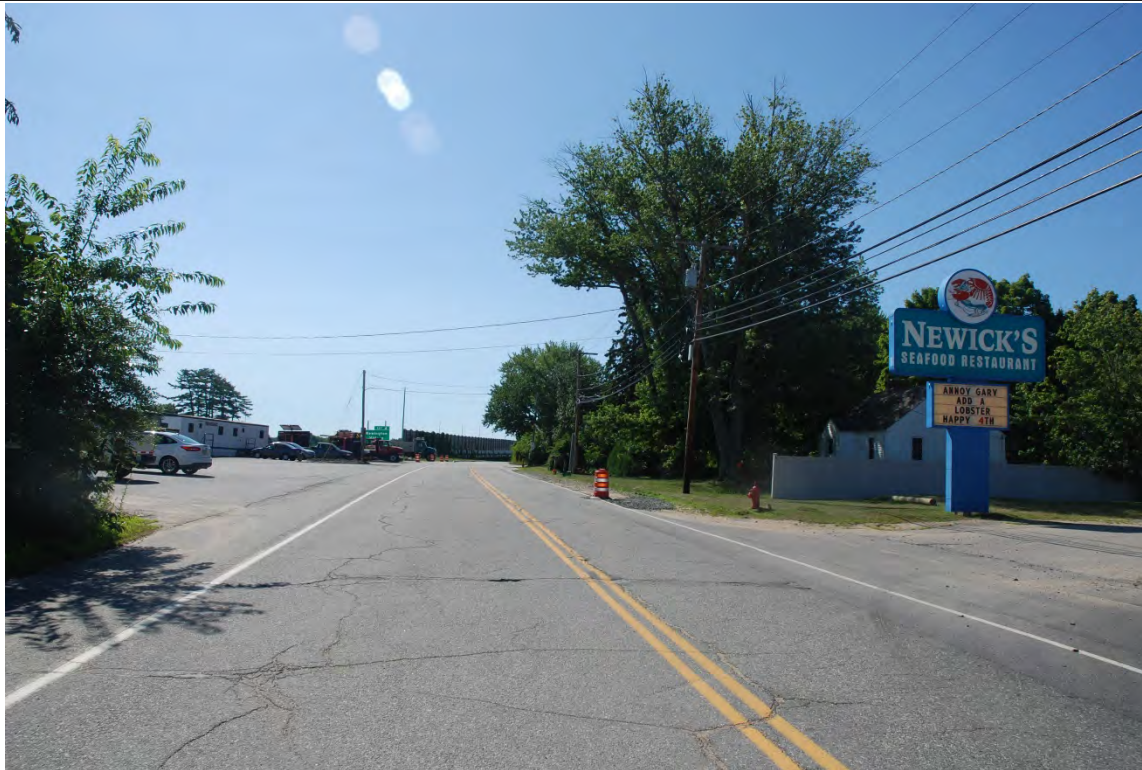
Photo # 1 Description: View along Dover Point Road, into project area
