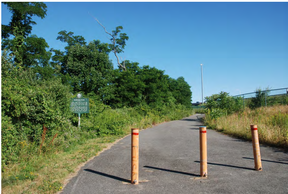
Photo # 26 Description: South approach to General Sullivan Bridge from Shattuck Way
