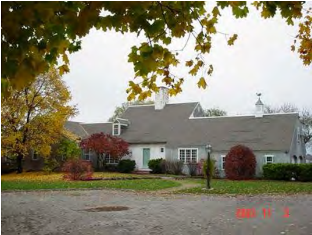
Photo # 43 Description: 137 Beane Lane (assessor's photo)
