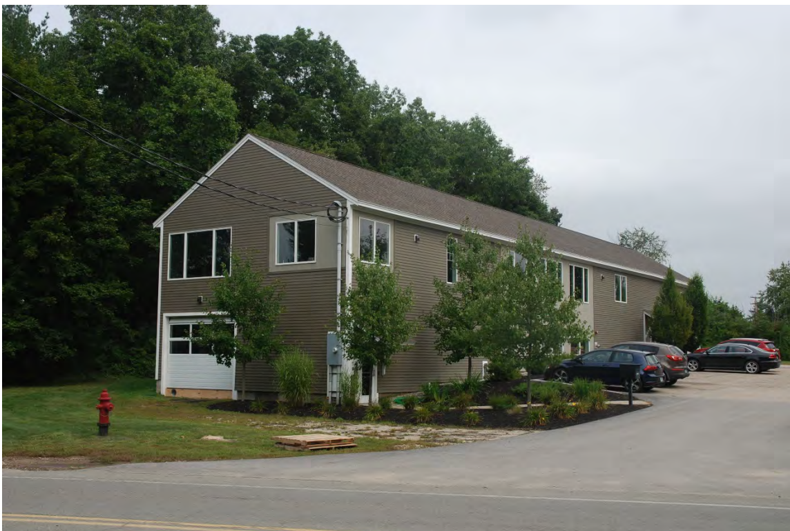
Photo # 38 Description: Atco LanAir Company, 521 Shattuck Way Reference (file name or frame #): 38_11238S Direction: NE
