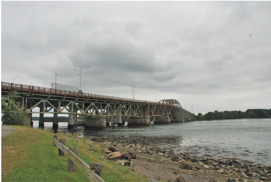
Photo # 25 Description: General Sullivan Bridge, DOV0158
