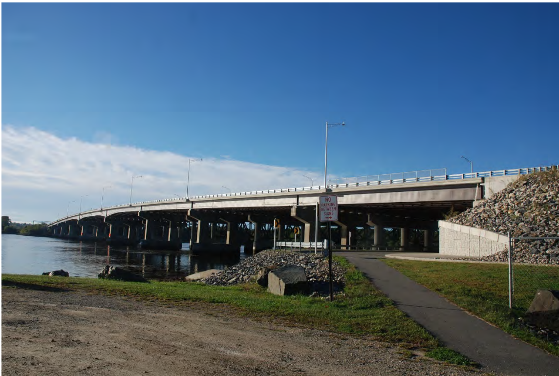
Photo # 24 Description: Little Bay Bridges Reference (file name or frame #): 24_11238S Direction: S Date: Sept. 2018
