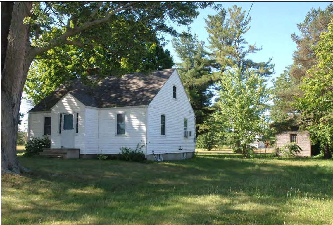
Photo # 3 Description: Belanger House, 435 Dover Point Road, DOV0092 Reference (file name or frame #): 3_11238S Direction: S
