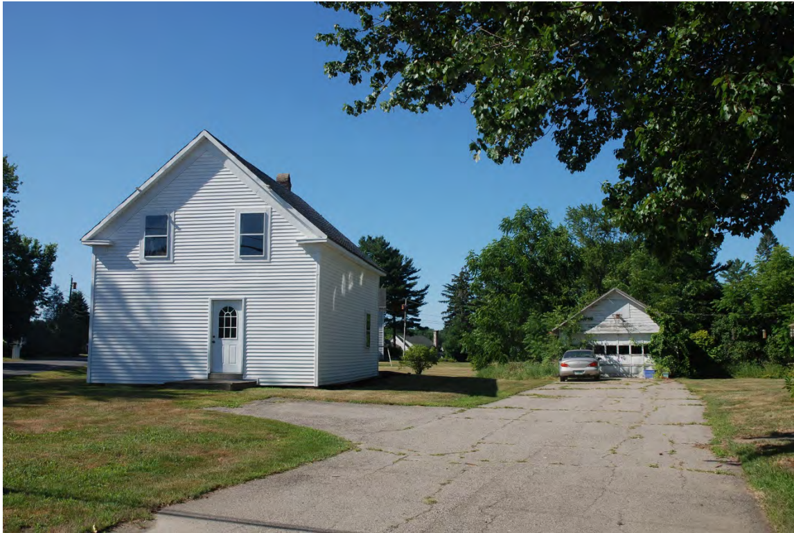
Photo # 7 Description: John E. Pinkham House (store and garage), 439 Dover Point Road, DOV0091 Reference (file name or frame #): 7_11238S Direction: SW Date: Aug. 2018
