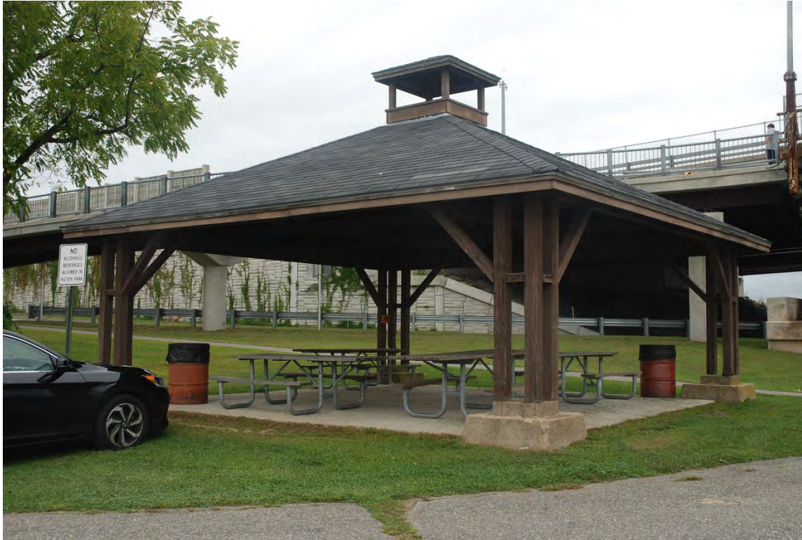
Photo # 21 Description: Hilton Park Roadside Safety Rest Area, DOV0150, picnic pavilion Reference (file name or frame #): 21_11238S Direction: N Date: Aug. 2018
