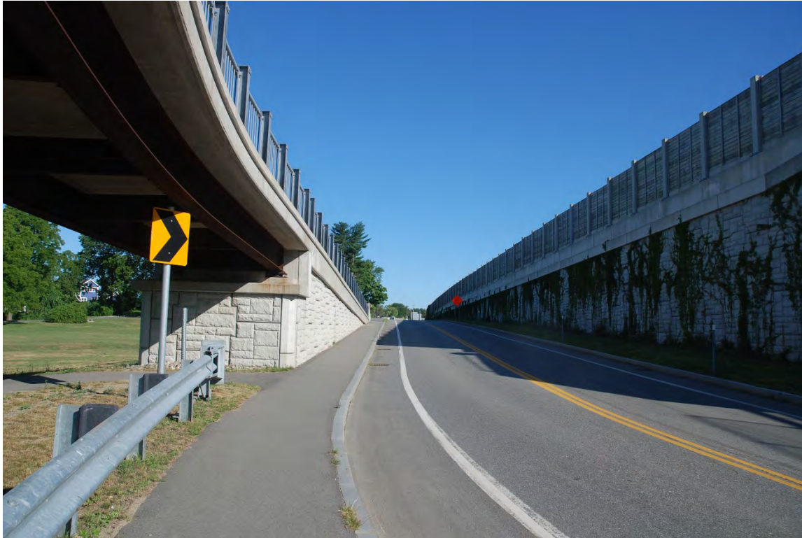
Photo # 19 Description: View along Hilton Park Road, approach ramp to General Sullivan Bridge on left, Spaulding Turnpike approach on right
